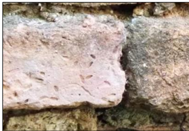
Fig.2 Brick with rice husks from Lulinkyaw gateway. (Photo: Field School of Archaeology - Pyay)
